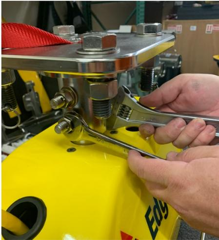
*Figure 4-49: 3400 Light and Ultra-Light Adaptor Flange Installation - Tightening Hardware Assembly*
